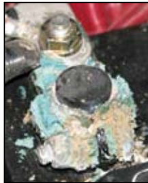
Battery terminal with corrosion build-up.
